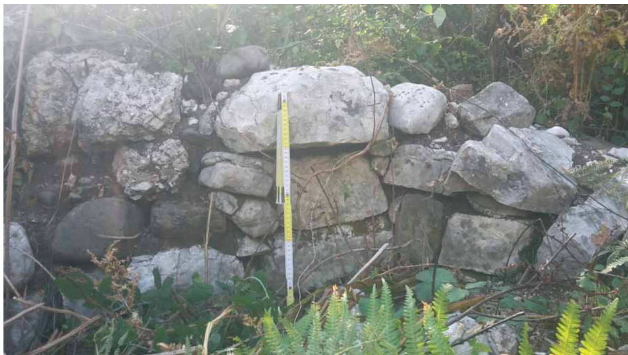
Fig. 14 — Terraced wall in the meander in Peshtan (photo: T. Rama)
