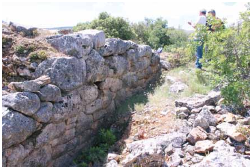
Fig. 14 – View of the central highest part of Z1 from the west side (photo: B. Kirigin)
