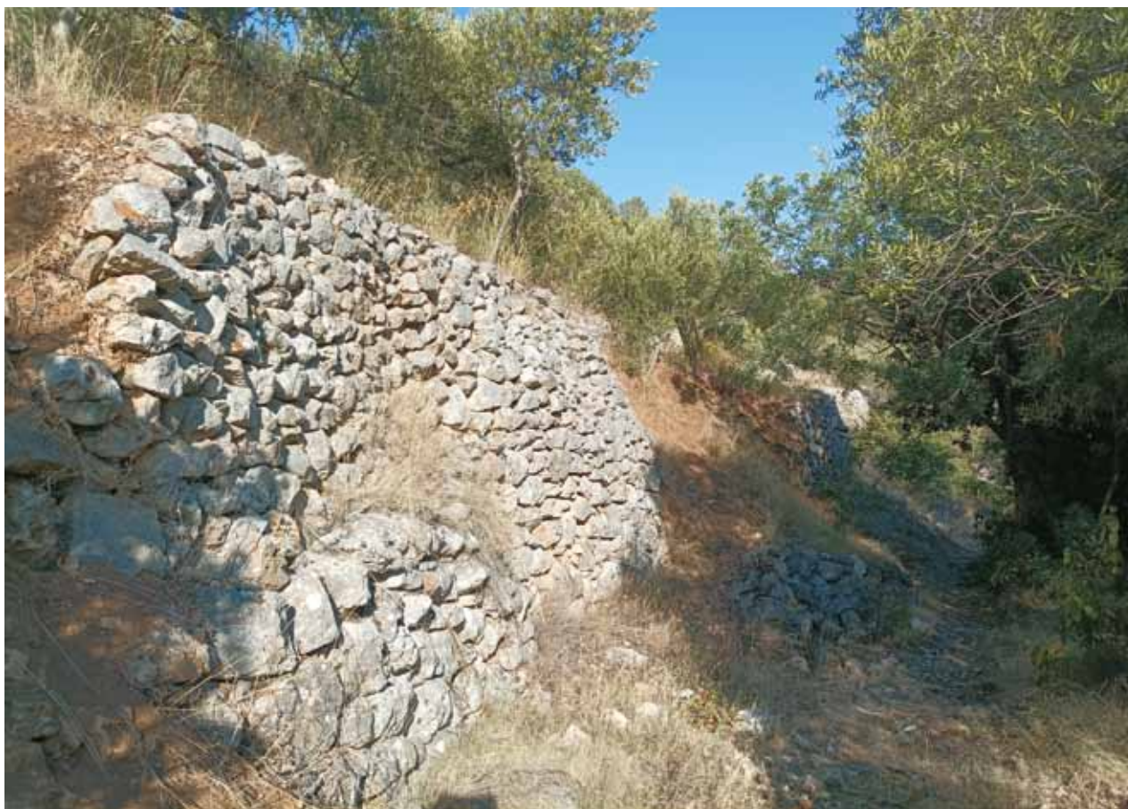
Fig. 32 – Tall dry stone wall (c. 3 m) along the paved path at the position of Laze (photo: B. Kirigin)
