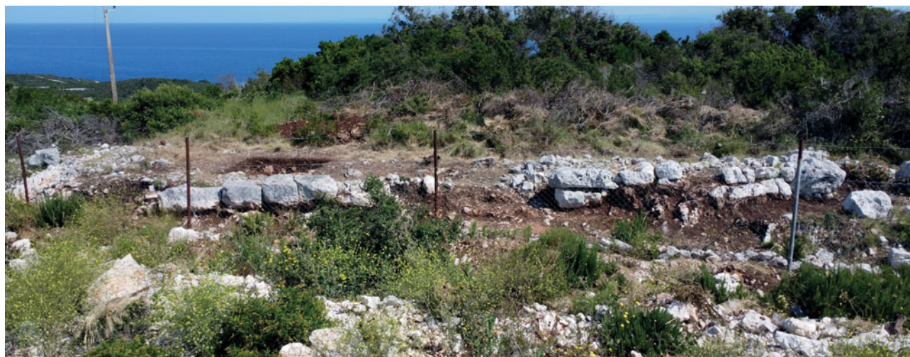
Sl. 3 Pogled na južno lice strukture (snimio: P. Domines Peter) Fig. 3 View of the southern face of the structure (photo by: P. Domines Peter)
