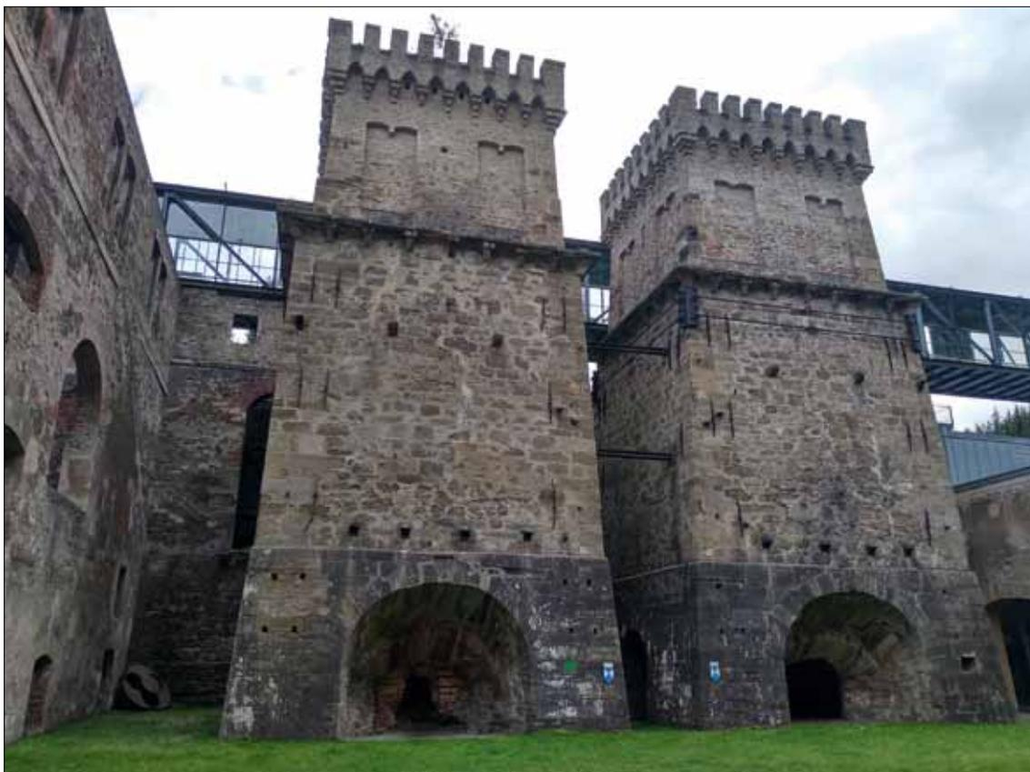
Fig. 4 Blast furnaces in Heft, near Hüttenberg, Carinthia. The building complex has been preserved from the mid-19<sup>th</sup> century (photo by: G. Oitzl)
