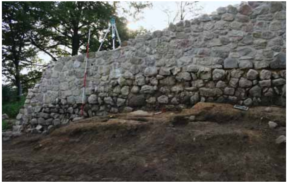
Fig. 31 A view from the west of the partially conserved wall SJ 62 and the remains of a timber structure
