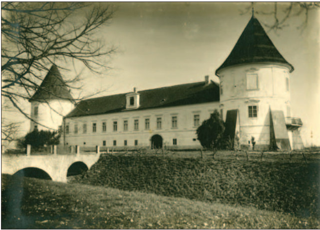
Fig. 11 Kerestinec mansion, northern façade (unknown author, end of 19 th c., Ministry of Culture, Directorate for the Protection of Cultural Heritage, Cultural heritage Documentation department, inv. no. 8487, neg. VII-232)
