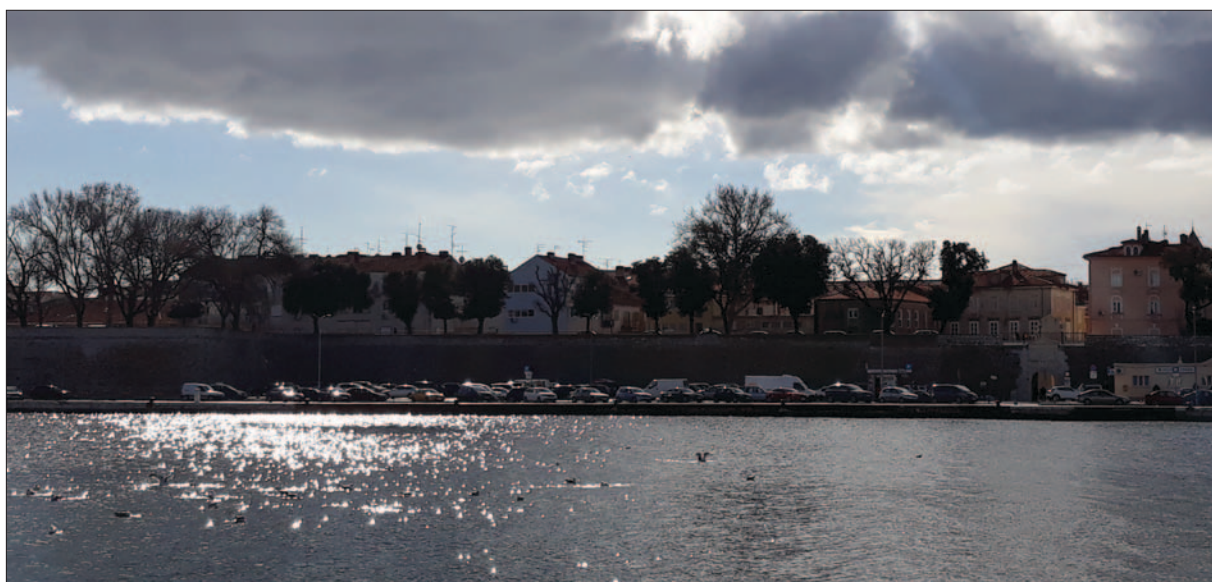
Fig. 5 Photography of the segment of the city walls on the port side, mentioned on a sketch from previous picture, on the right – Porta Marina, on the opposite left – Bastion Wagner (photo by: D. Štrmelj)
