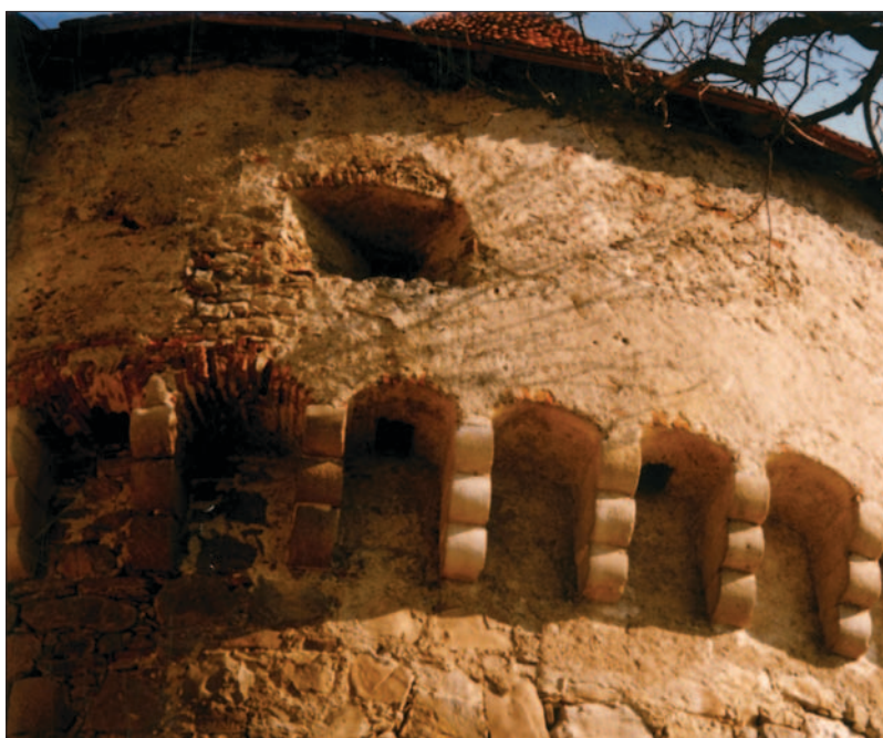
Fig. 43 Veliki Tabor castle: superstructure supported by corbels around the whole fort (photo by: Z. Horvat)
