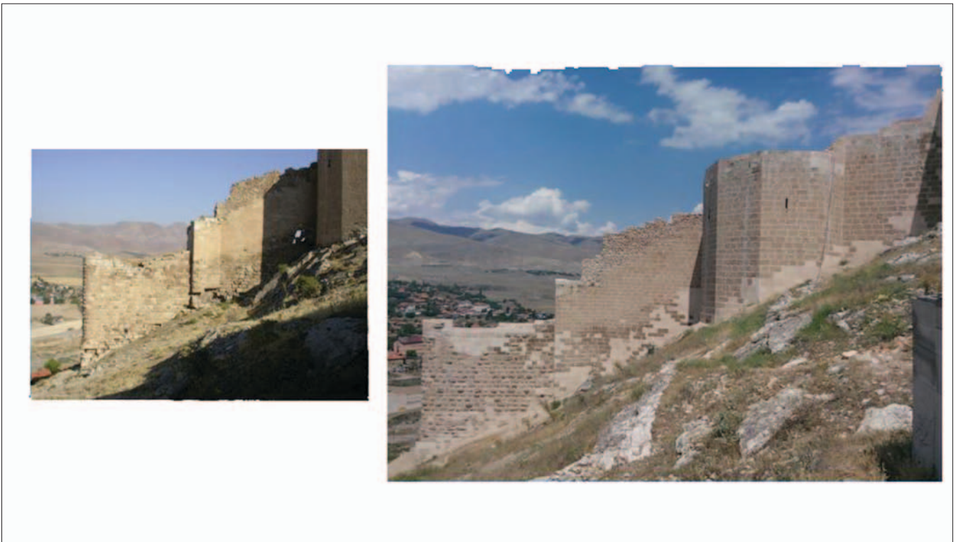
Fig. 14 South wall before and after the restoration (photos by: E. Eser, 2017)
