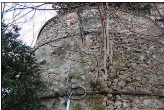
Fig. 2 The tower of the town walls on the north side of the castle: view from below (photo by: C. Mazzanti 2015)
