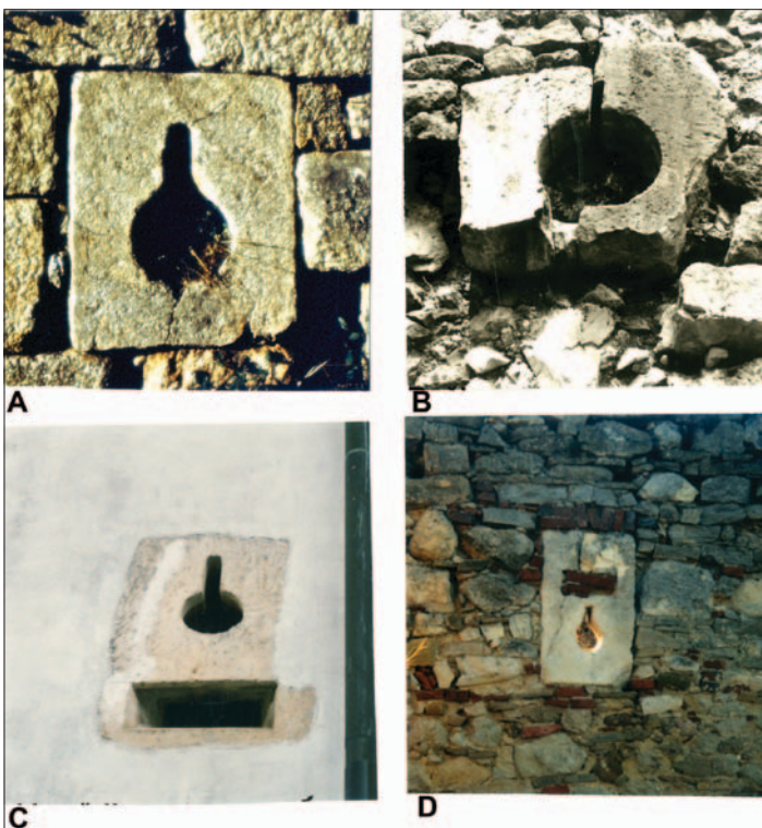
Fig. 23 Gun loop openings: A – Brinje, B - Ružica, western wall, C – Stari grad Varaždin, D – Konjščina (photo by: Z. Horvat)
