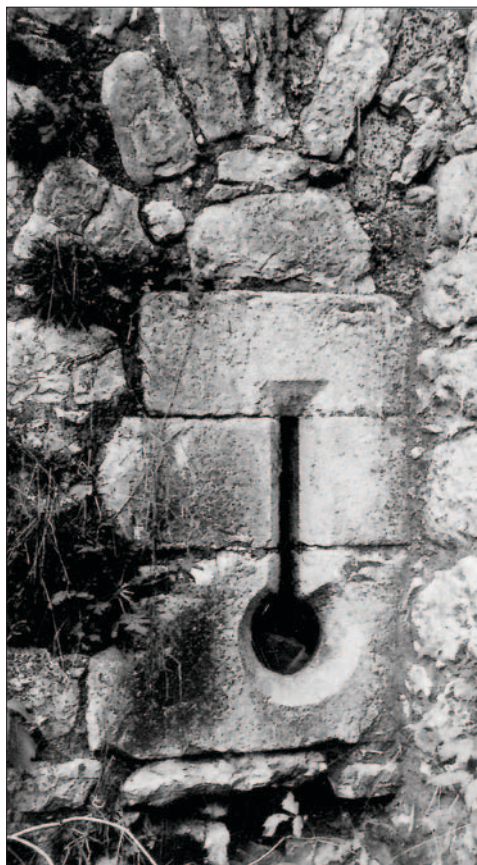
Fig. 17 Ribnik castle near Karlovac from the second half of the 15 th century: cross-bow slit next to a pentagonal tower, view from the outside (photo by: Z. Horvat)
