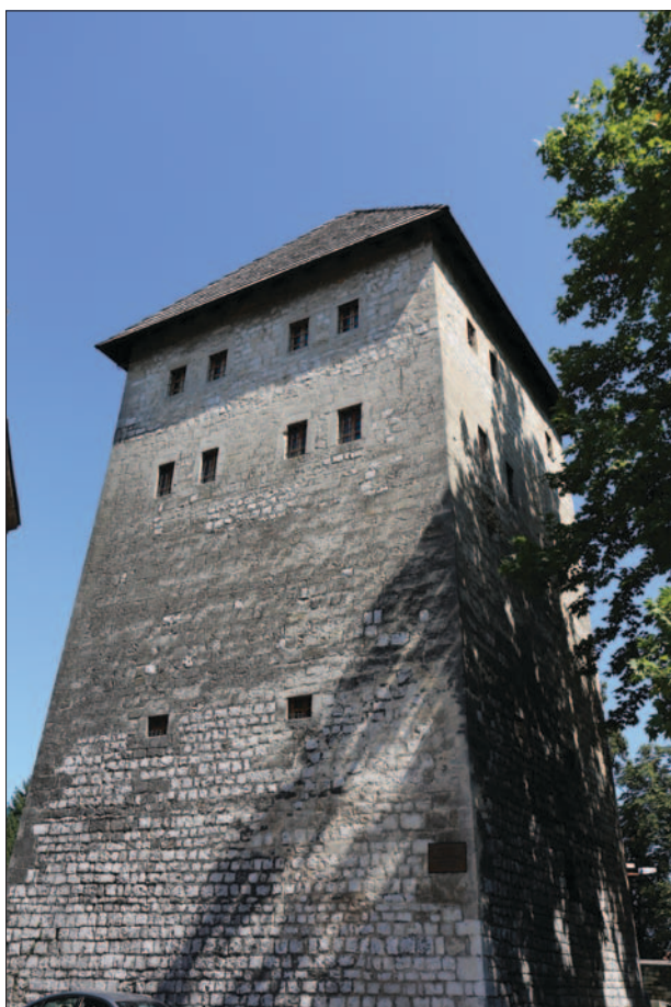
Fig. 15 Bihać – view on tower near city wall (photo by M. Procházka)
