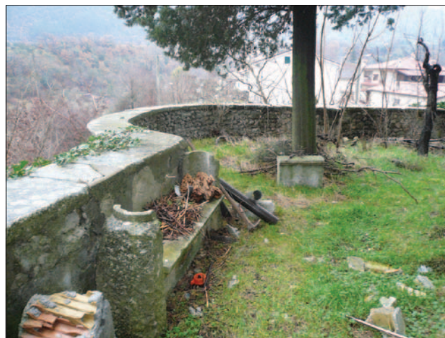
Fig. 3 The tower of the town walls on the north side of the castle: view from the stands (photo by: C. Mazzanti 2015)
