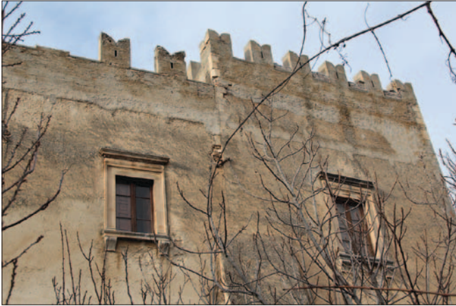
Fig. 7 The Cantelmos Castle of Bussi: detail of the south façade (photo by: C. Mazzanti 2015)
