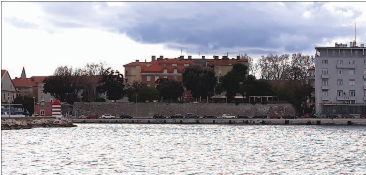
Fig. 3 Photography of the Bastion della Sanita today (photo by: D. Štrmelj)
