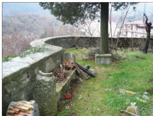
Fig. 3 The tower of the town walls on the north side of the castle: view from the stands (photo by: C. Mazzanti 2015)
