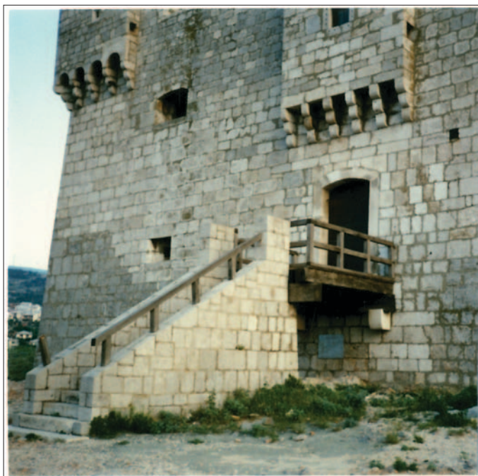
Fig. 42 Senj, Nehaj castle (mid-16 th century): bay window above the entrance (photo by: T. Petrinec)
