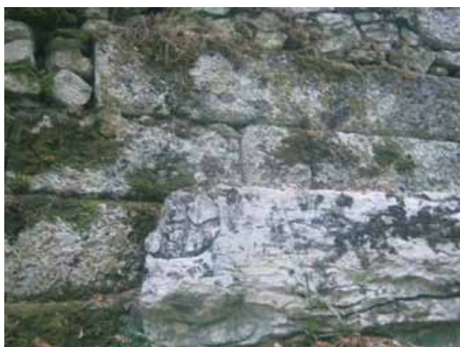
Fig. 11 — Sections of the blocking wall (photo: T. Rama)
