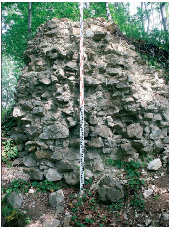
Sl. 13 Zid uz branič-kulu (snimio J. Belaj) Fig. 13 The wall next to the defensive tower (photo by J. Belaj)
