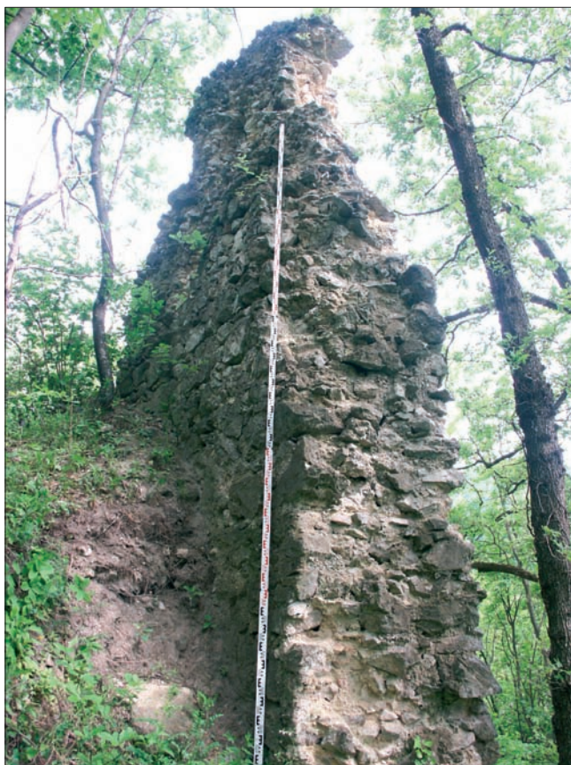
Sl. 8 Ostatak južnog zida, unutarnja strana (snimio J. Belaj) Fig. 8 The remains of the southern wall, the interior (photo by J. Belaj)
