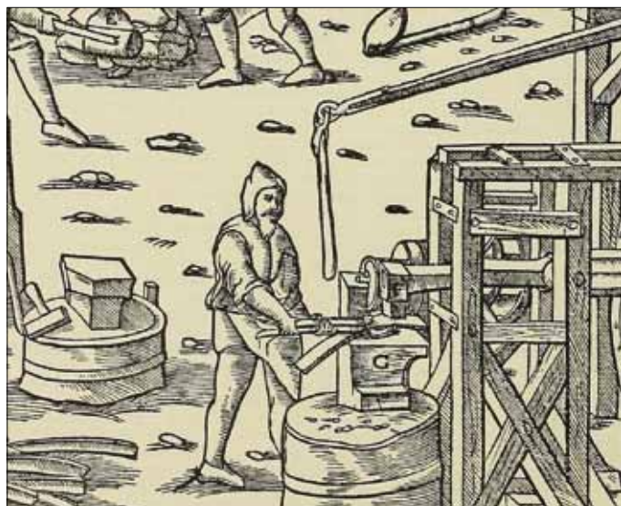
Fig. 1 A detail of a mid-16 th -century woodcut showing the use of a water-powered hammer to process iron (Georg Agricola, De re Metallica , © archive.org)
