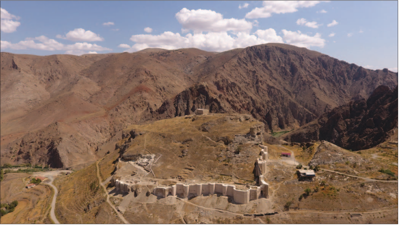
Fig. 16 Aerial view of the Divriği castle after the finished first phase of the restoration (photo by: O. Tecer, 2017)
