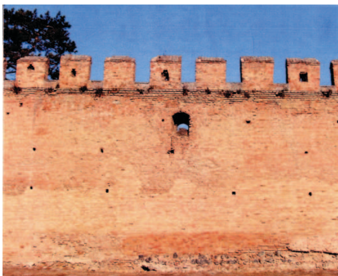
Fig. 11 Ilok, part of the northern wall (photo by: Z. Horvat)
