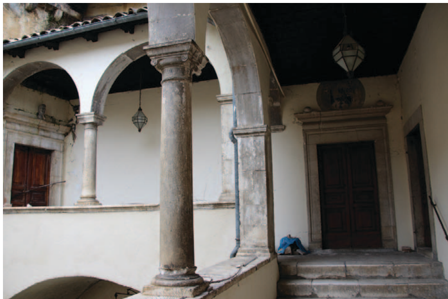
Fig. 6 The Cantemos Castle of Bussi: view of the internal courtyard (photo by: C. Mazzanti 2015)
