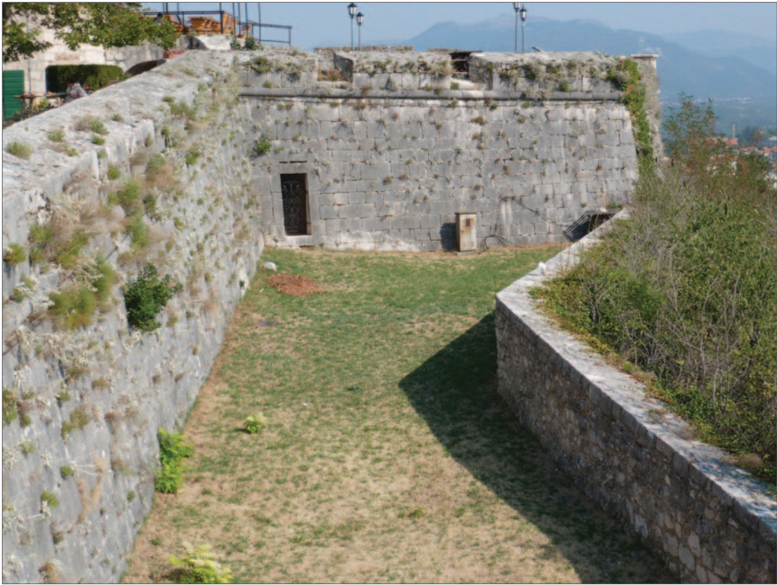
Fig. 4 Knin, bastion Pisani and falsabragha (photo by: A. Žmegač)
