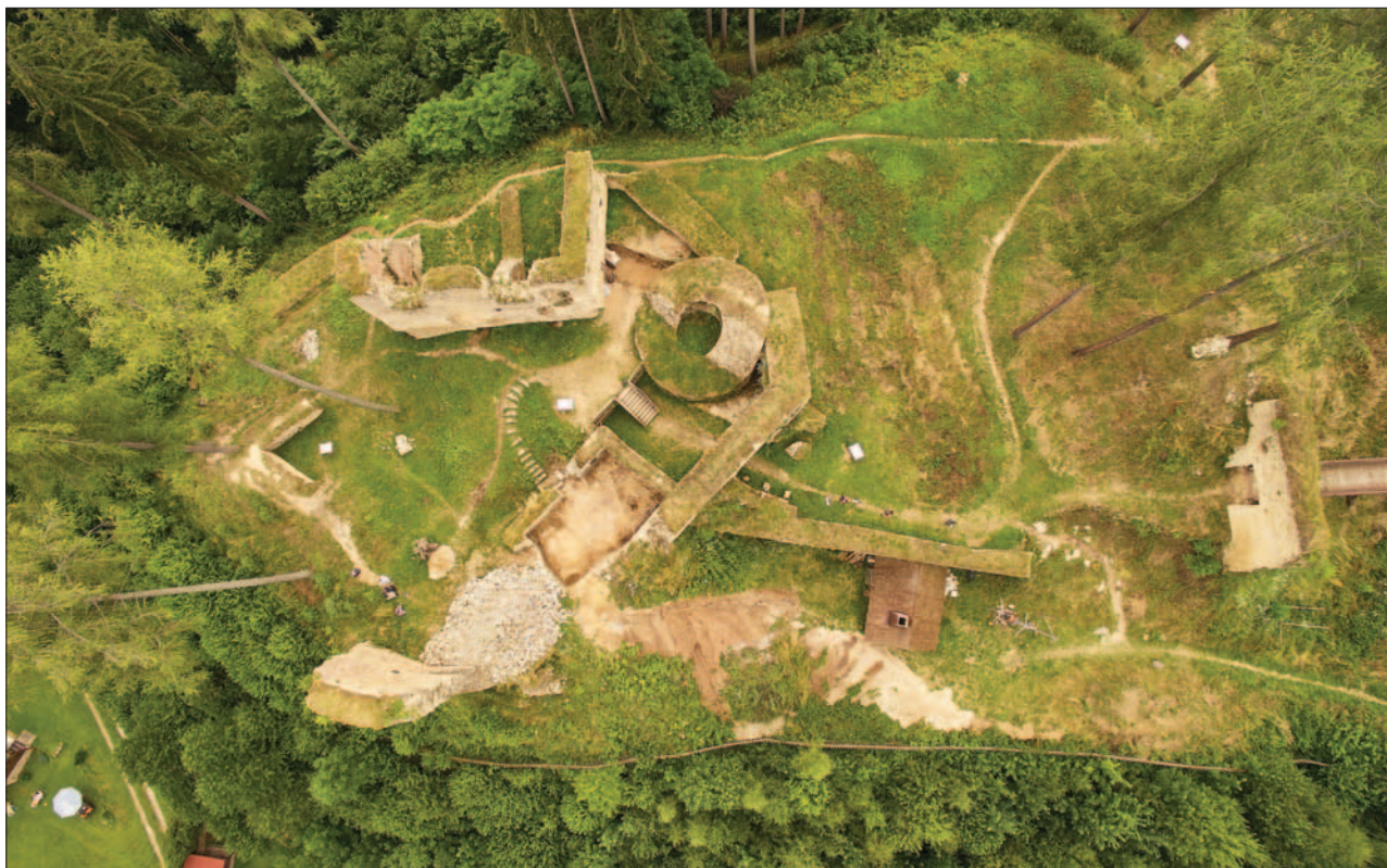
Fig. 10 Pořešín castle: aerial photo of central castle (photo by: J. Hložek)
