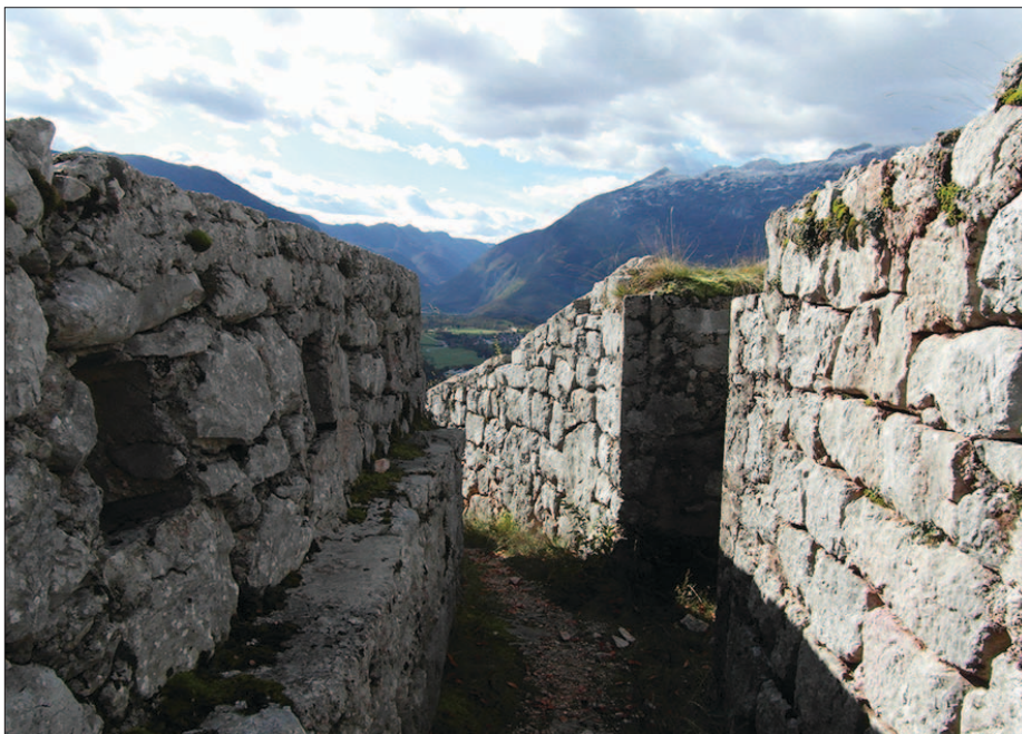
Fig. 3 Stone built trench with embrasures at Stützpunkt Kal, today's Čelo (650 m) above Kal-Koritnica village (photo by: U. Košir, 2014)
