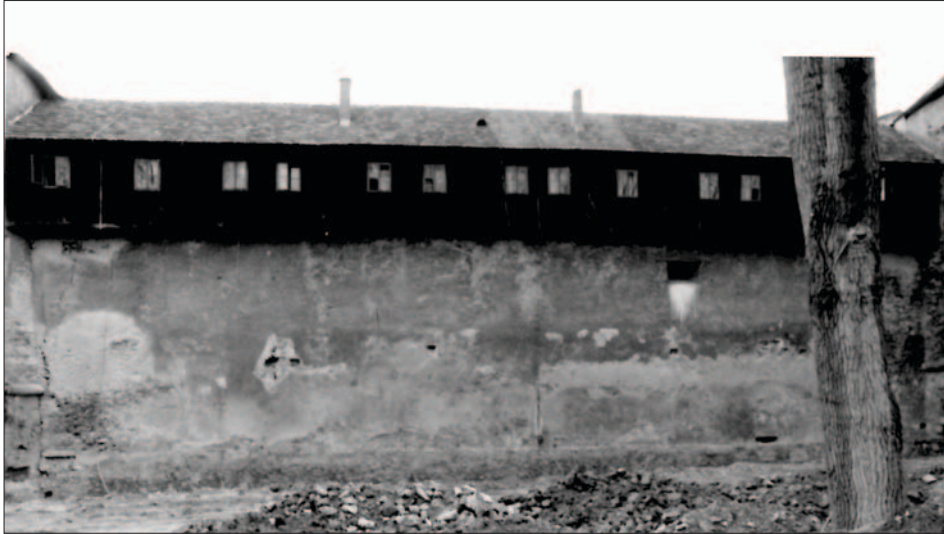
Fig. 39 Sisak castle, top of the walls with a wooden construction, current state (photo by: J. Škudar, Croatian Conservation Institute)
