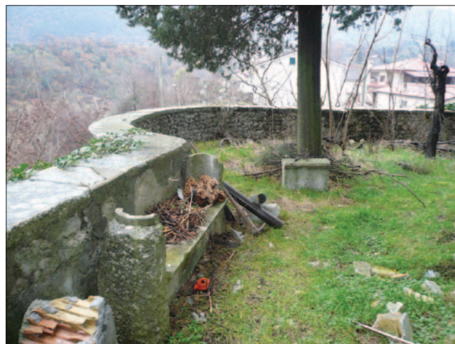
Fig. 3 The tower of the town walls on the north side of the castle: view from the stands (photo by: C. Mazzanti 2015)
