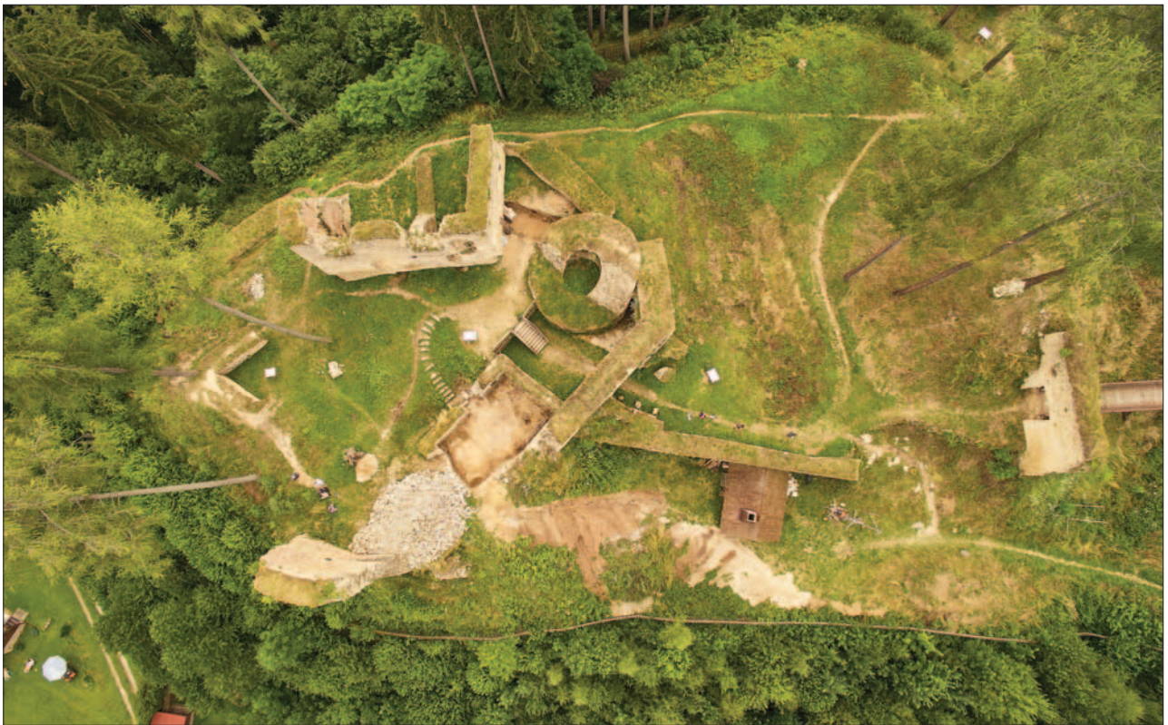
Fig. 10 Pořešín castle: aerial photo of central castle (photo by: J. Hložek)
