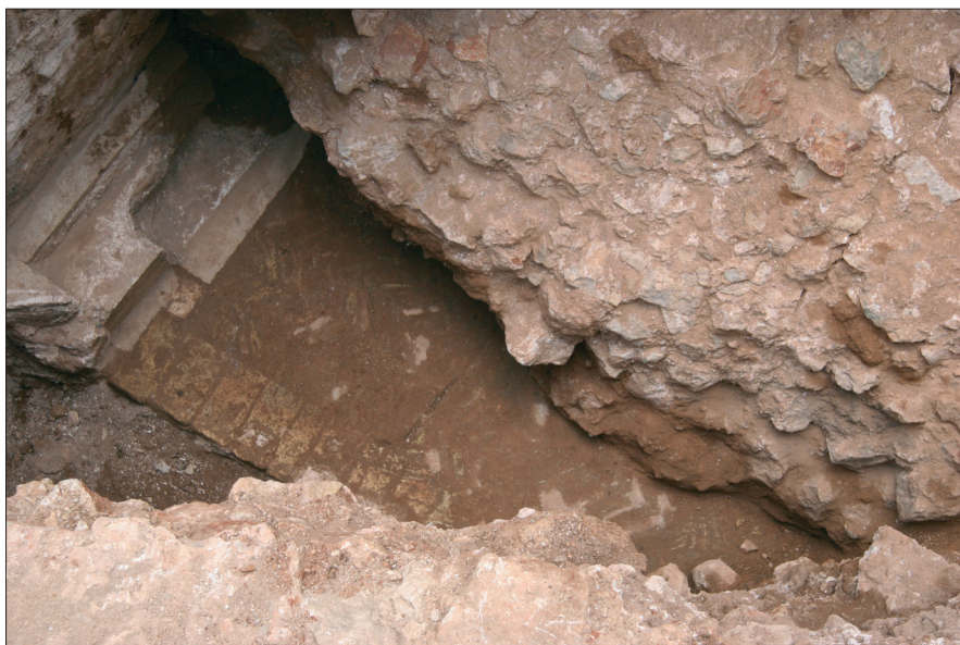
Fig. 6 Remains of the treading surface of John of Sienna Bridge (photo by: Ž. Peković)
