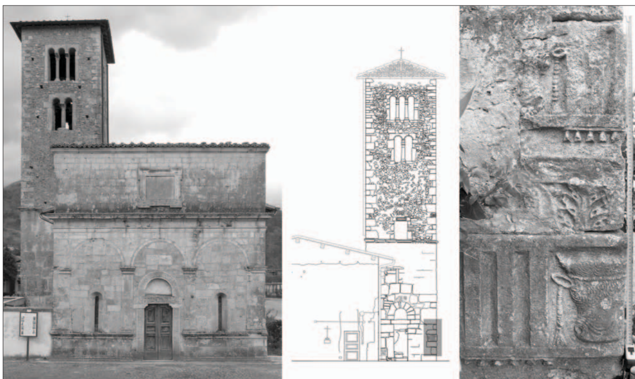
Fig. 1 Carsoli, reuse elements at the base of the bell tower of the church of Santa Maria in Cellis (drawing and graphic elaboration by: S. Cecamore, 2011)
