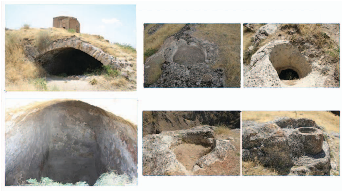
Fig. 5 Blood pits and cistern in the north area of the castle (photo by: E. Eser, 2016)
