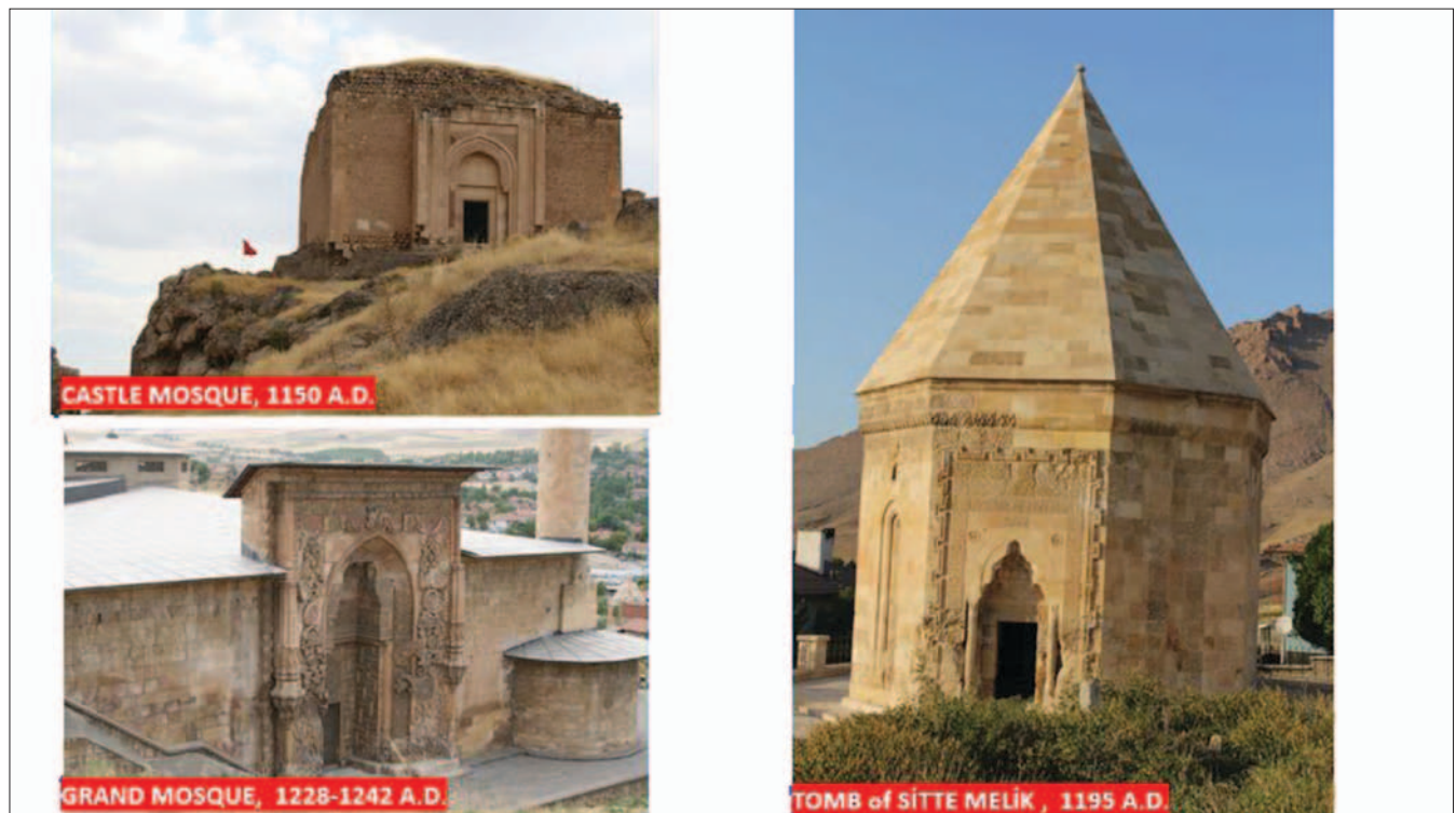
Fig. 10 Photographs of the buildings from Mengücek period in Divriği (photos by: E. Eser, 2014)
