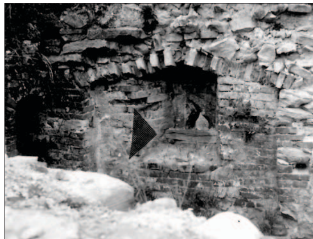
Fig. 20 Konjščina castle, partially preserved gun loop on the 1 st floor of the gatehouse: notice the wooden beam along the outer opening of the gun loop (photo by: Z. Horvat)
