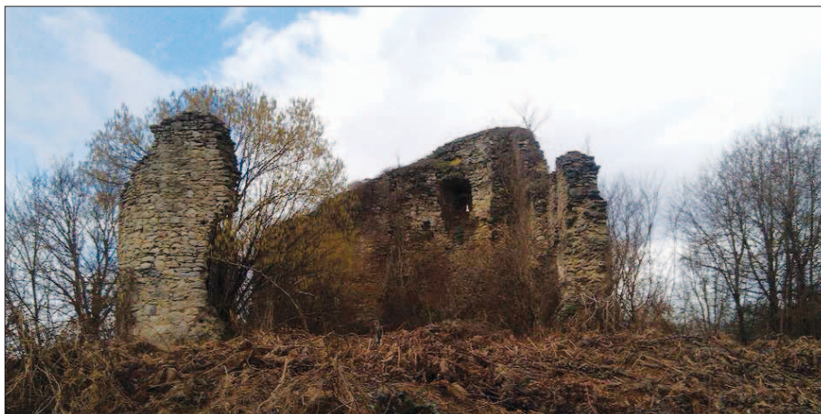
Fig. 9 Klokoč, southeastern corner (photo by: Višnja Bedenko)
