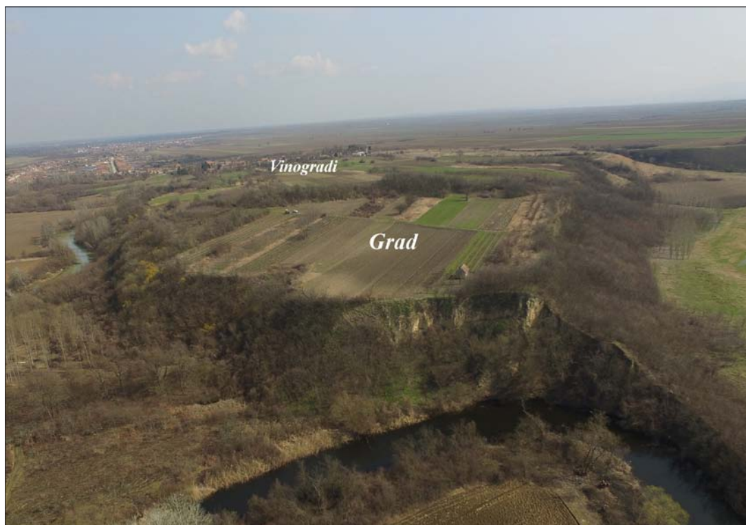
Fig. 9 Dupljaja, medieval fortress, aerial view from the west (photo by: D. Radičević)
