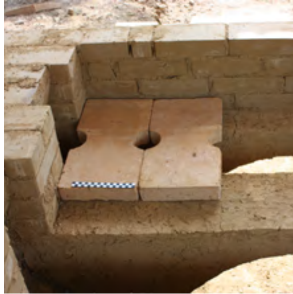
Sl. 15 Ploče (opeke) s polukružnim bočnim otvorima koje čine dio rešetke. Položene su na lukove mostova (foto: A. Konestra) Fig. 15 Slabs (bricks) with semicircular side apertures which form a part of the grid. They are set upon the arches of the bridges (photo: A. Konestra)
