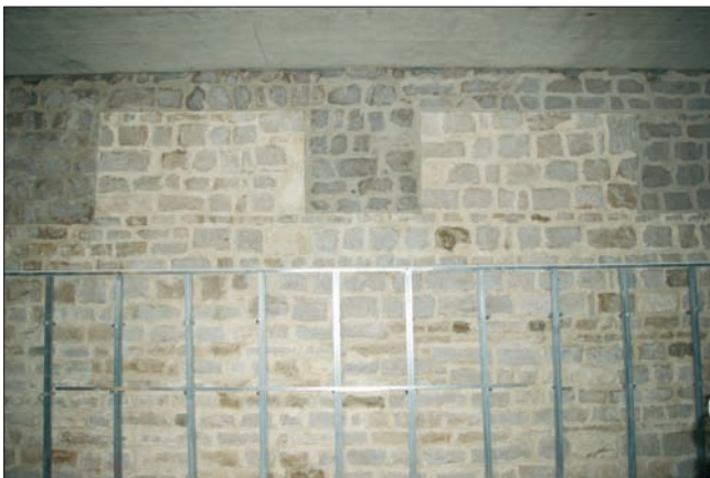
Sl. 11 Obrisi kruništa na istočnom zidu Citadela Fig. 11 Outlines of the battlement on the eastern wall of the Citadela
