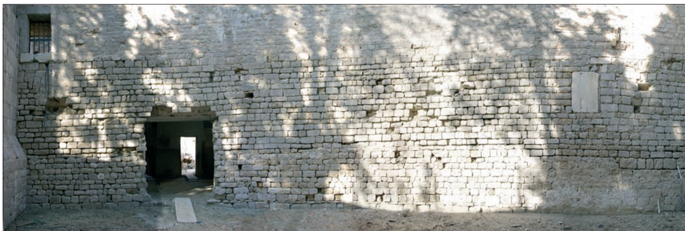
Sl. 10 Istočni zid Citadela Fig. 10 Eastern wall of the Citadela
