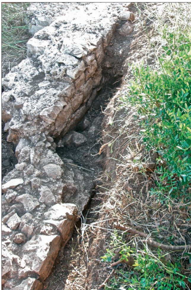
Sl. 6 Zid ranocarske vile (snimio: T. Schrunk) Fig. 6 Wall of the Early Imperial villa (photo: T. Schrunk)
