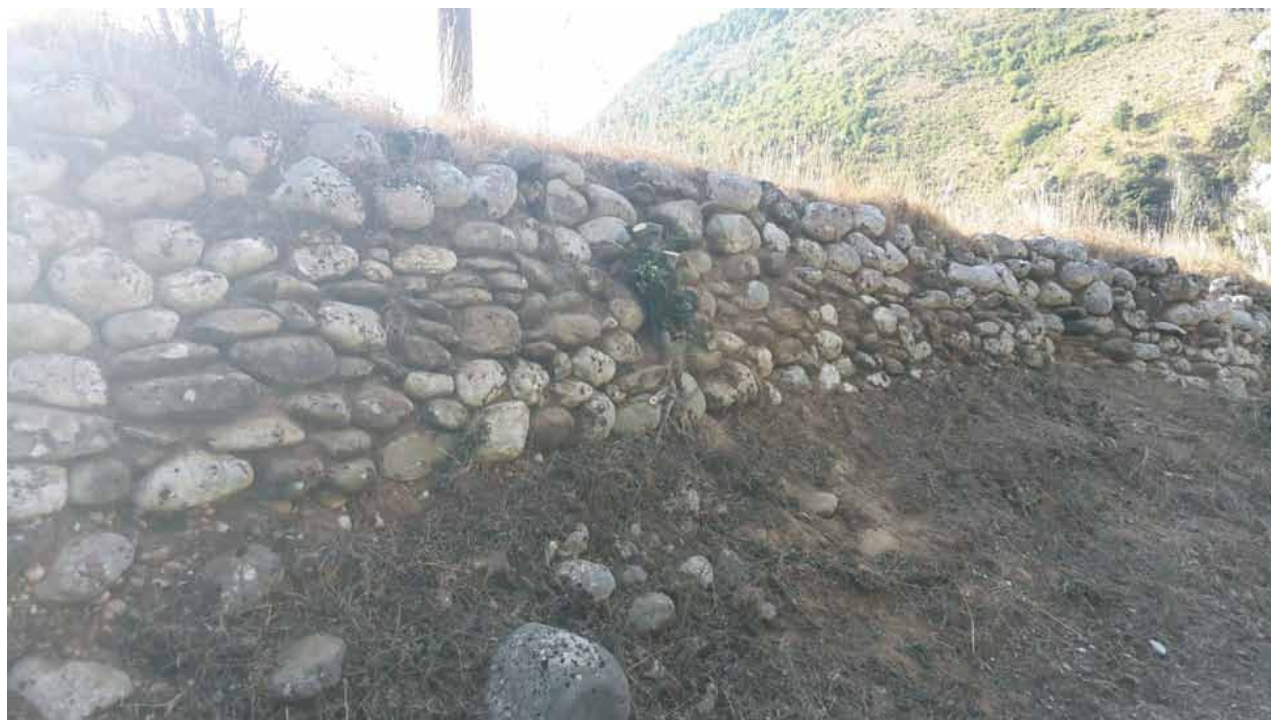
Fig. 15 — Terraced wall in the meander in Peshtan (photo: T. Rama)
