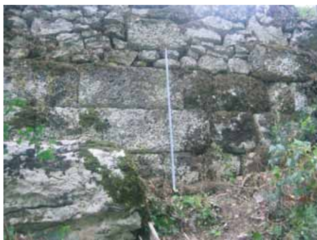
Fig. 12 — Sections of the blocking wall (photo: T. Rama)
