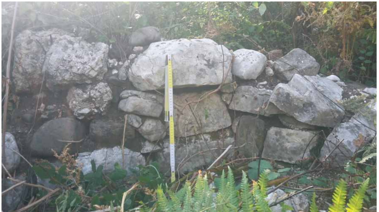
Fig. 14 — Terraced wall in the meander in Peshtan (photo: T. Rama)
