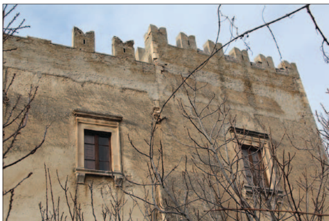
Fig. 7 The Cantelmos Castle of Bussi: detail of the south façade (photo by: C. Mazzanti 2015)
