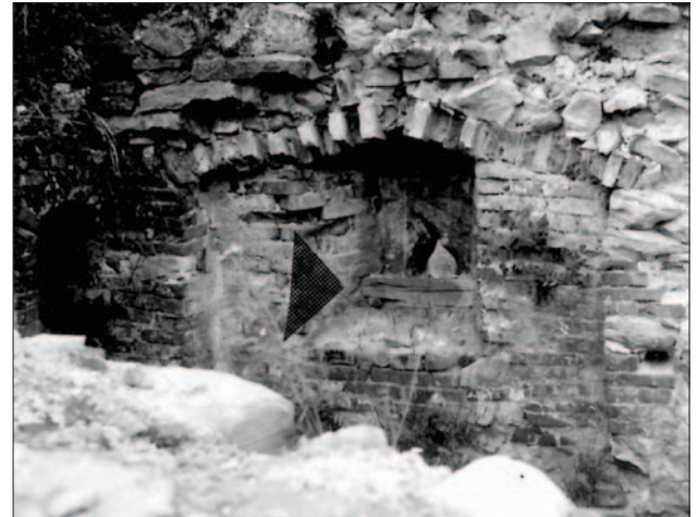
Fig. 20 Konjščina castle, partially preserved gun loop on the 1 st floor of the gatehouse: notice the wooden beam along the outer opening of the gun loop (photo by: Z. Horvat)
