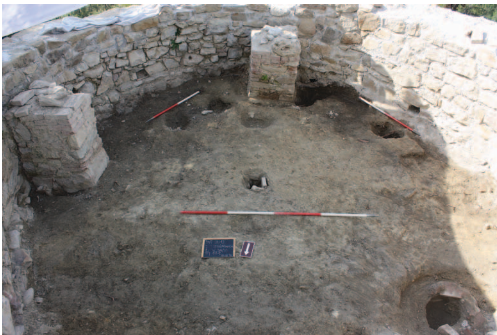
Fig. 16 Veliki Tabor castle – round south circular tower of outer defence wall, screed floor that functioned with massive square-shaped masonry bases/supports (Photo Library of Museums of Croatian Zagorje – Veliki Tabor Castle)
