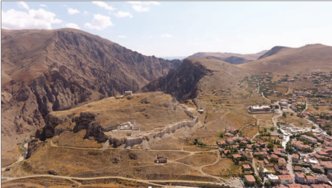
Fig. 3 Aerial view of Divriği castle from the Northwest (photo by: O. Tecer, 2017)
