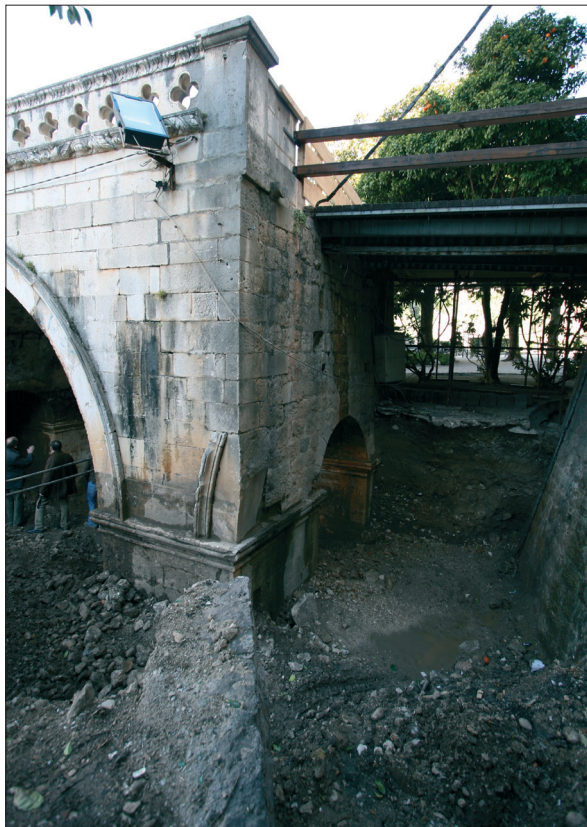
Fig. 11 Traces of the third arch on Paskoje's bridge (photo by: Ž. Peković)
