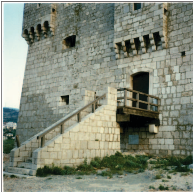
Fig. 42 Senj, Nehaj castle (mid-16 th century): bay window above the entrance (photo by: T. Petrinec)
