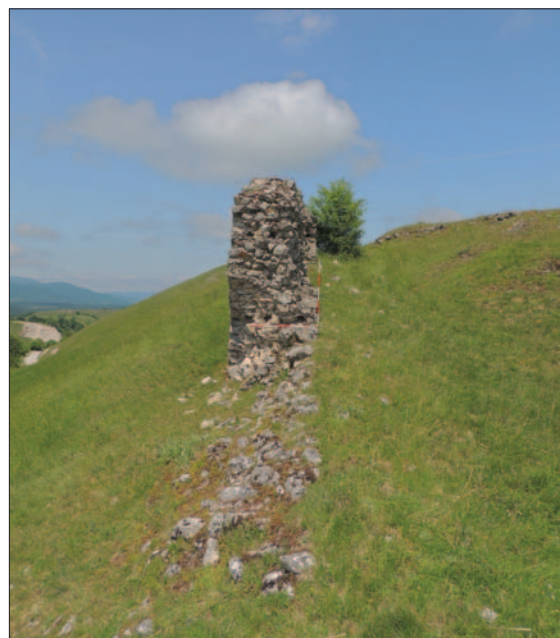
Fig. 4 Bjelaj – remains of wall in bailey (photo by: M. Procházka)
