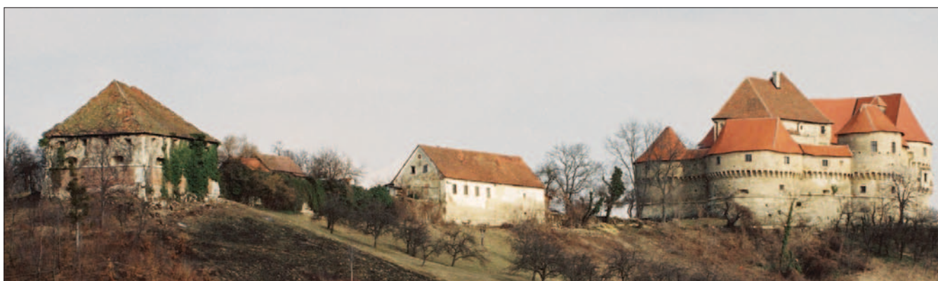
Fig. 7 Veliki Tabor complex before renovation (Photo Library of Museums of Croatian Zagorje – Veliki Tabor Castle)
