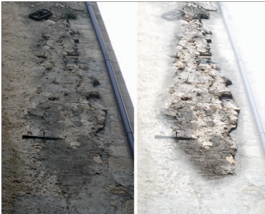
Fig. 4 The Cantelmos Castle of Bussi: detail of the west front and highlight of the remains of the initially fortified structure (picture by: C. Mazzanti 2015)
