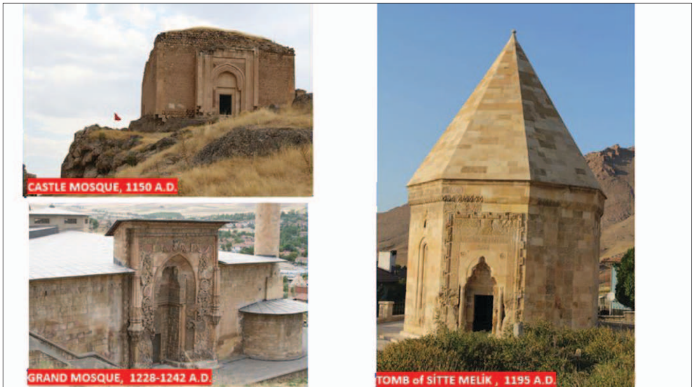
Fig. 10 Photographs of the buildings from Mengücek period in Divriği (photos by: E. Eser, 2014)
