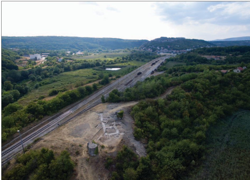
Fig. 7 The Kapitul viewed from the south with the fort of Knin on the hill Spas in the background (photo by: Z. Tanocki, 2016)
