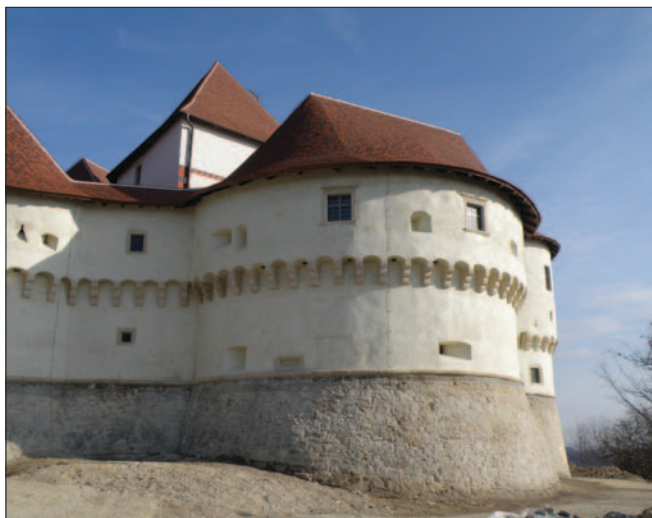
Fig. 5 Veliki Tabor castle – southwest Renaissance semi-circular tower (Photo Library of Museums of Croatian Zagorje – Veliki Tabor Castle)
