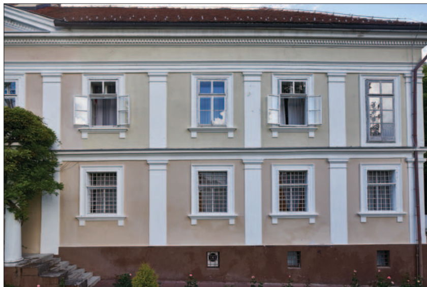
Fig. 5 Bežanec mansion, segment of southeastern façade (photo by: Jasenko Rasol, 2016)
