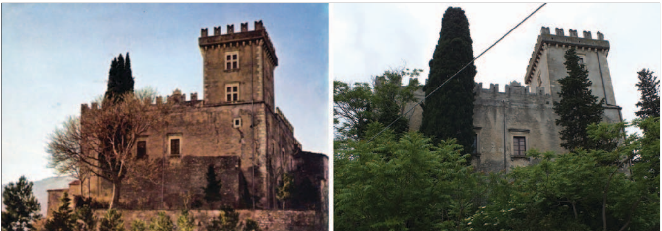
Fig. 5 The Cantelmos Castle of Bussi: view of the mid-20 th century (Municipal Historical Archive of Bussi) and current view (photo by: C. Mazzanti 2015)
