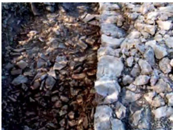
Fig. 8 Part of the western wall of the castellum with tegulae fallen from the roof of the adjacent portico Sl. 8 Dio zapadnog zida castelluma s tegulama palim s krova obližnjeg portika
