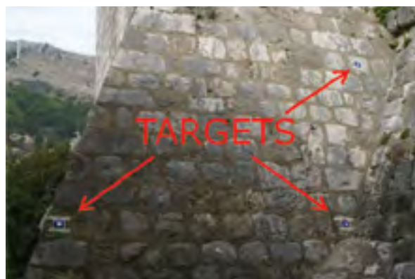
Fig. 2 Marks (targets) on the object of scanning Sl. 2 Oznake (mete) na objektu skeniranja
