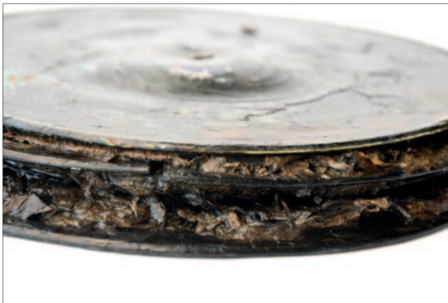
Sl. 9 Slojevi slame među prozorskim staklima, 2020. (snimio: M. Martinčak) Fig. 9 Layers of straw between window panes, 2020 (photo by: M. Martinčak)
